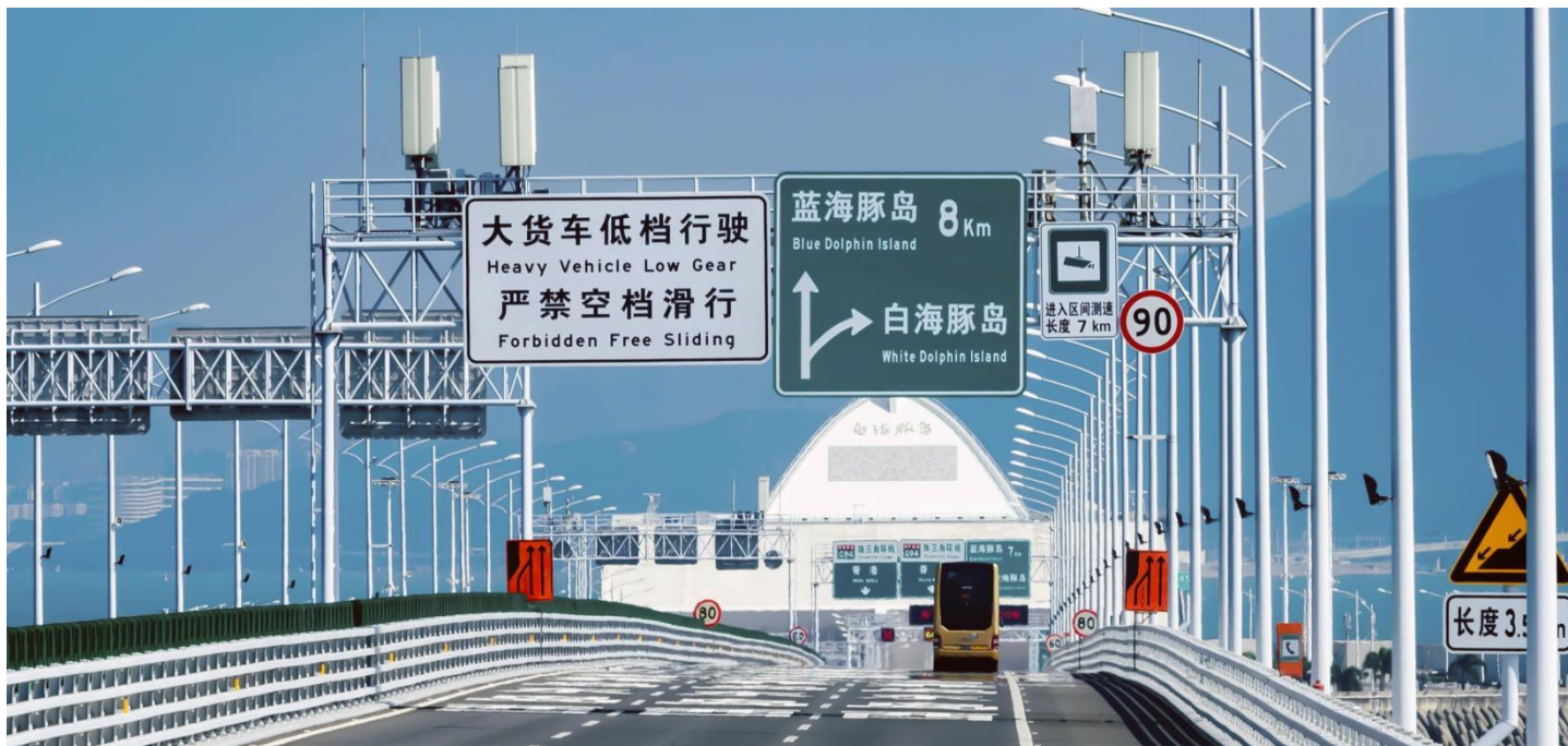
KBT Antennas Deployed at Hong Kong-Zhuhai-Macao Bridge
